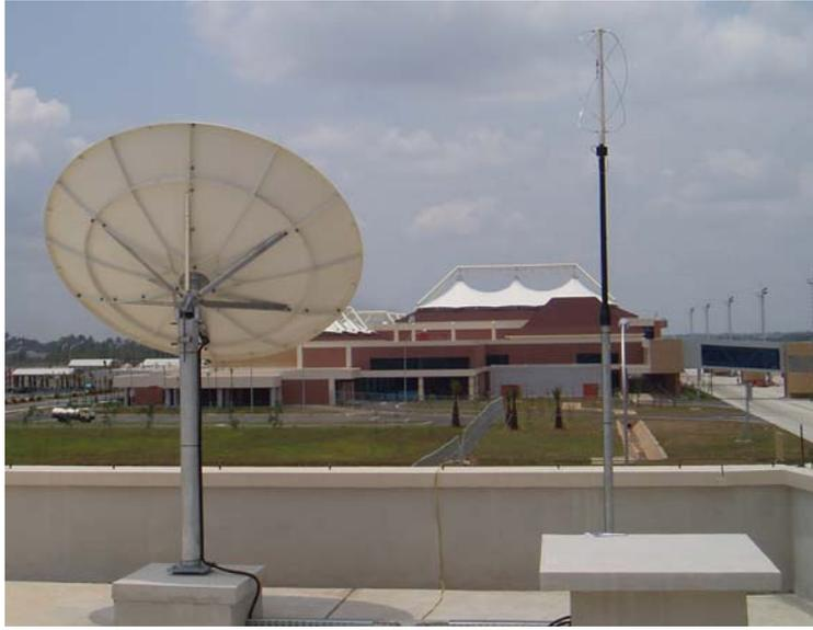
Satellite dish and WEFAX antenna installation for weather satellite imagery. Allows a link to Asian weather satellites and delivers weather imagery to all workstations and displays attached to the system.
